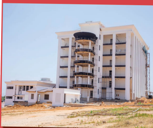
Viwango House under construction at Njedengwa, Dodoma
